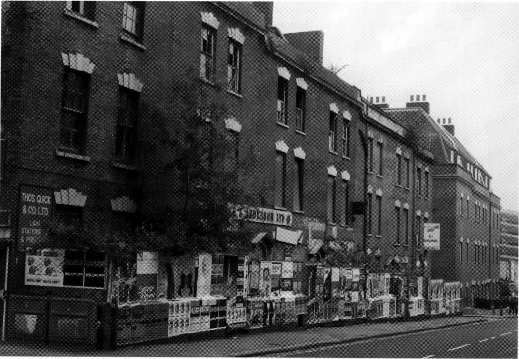
Fig. 6 Nos 1-13 St Paul's Street, Bristol
